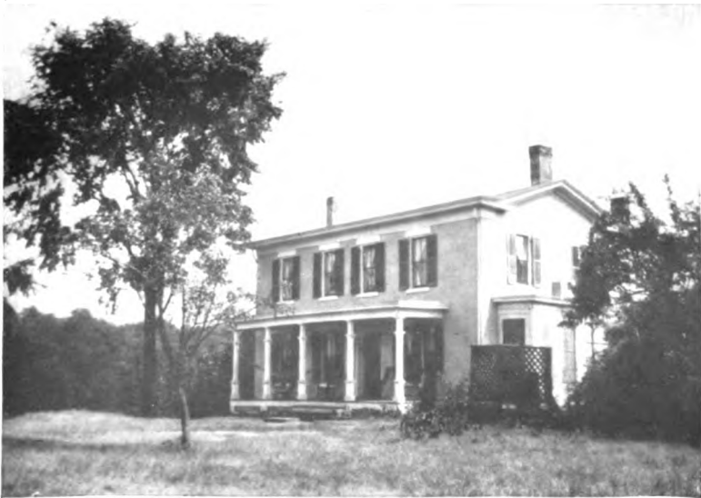
The Francis Pruyn-Davie Homestead From a photograph
