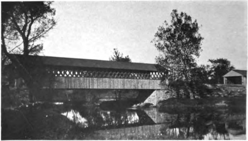
The Village Bridges
